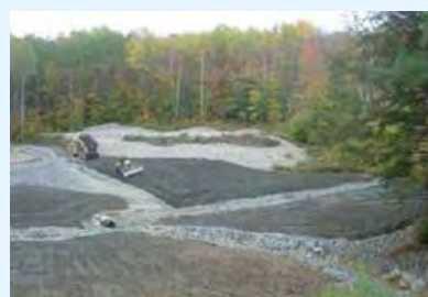
Designs for backfilling, grading and stabilizing a 3-acre basin affected by mining waste at the Elizabeth Mine NPL site in South Strafford, Vermont, included intent to mirror the site's natural contours and drainage patterns. The fully graded surfaces were seeded with native plant species that target Vermont state conservation and wildlife goals.
