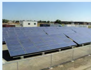
Operation of photovoltaic systems at the Frontier Fertilizer Superfund site in Davis, California, avoids an estimated 147,500 pounds in CO 2 (equivalent) emissions each year. The systems involve a ground-mounted solar array as well as a roof-mounted solar array that together offset 100 percent of the grid electricity used to pump and treat the site's contaminated groundwater. 29
